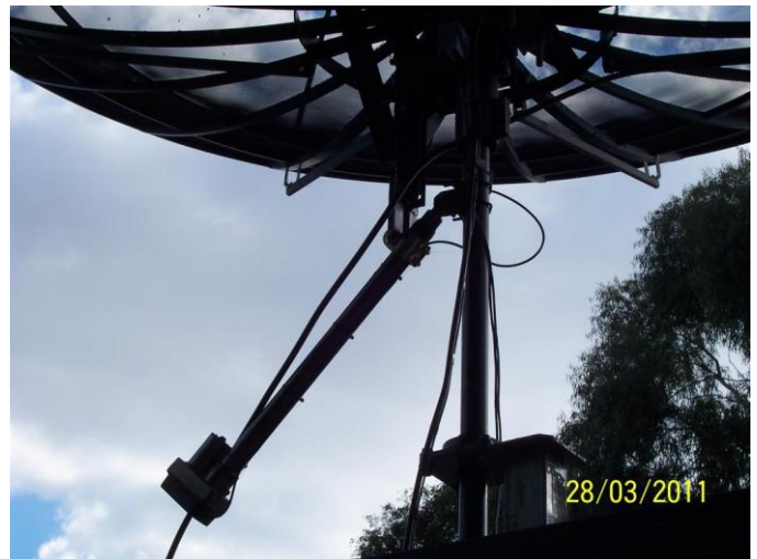
Screw Jack for driving Elevation
